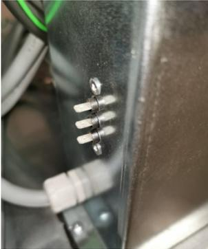
These units are equipped with remote alarm terminals for the connection to a remote alarm network.
