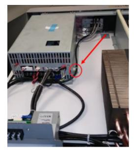
Note: Disconnect all electrical clip connections to the power supply and the ground wire nut as shown. Make sure not to remove power receptacle harness.
